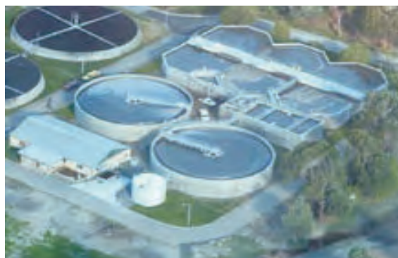
Figure 8.7 An aerial view of a sewage plant
